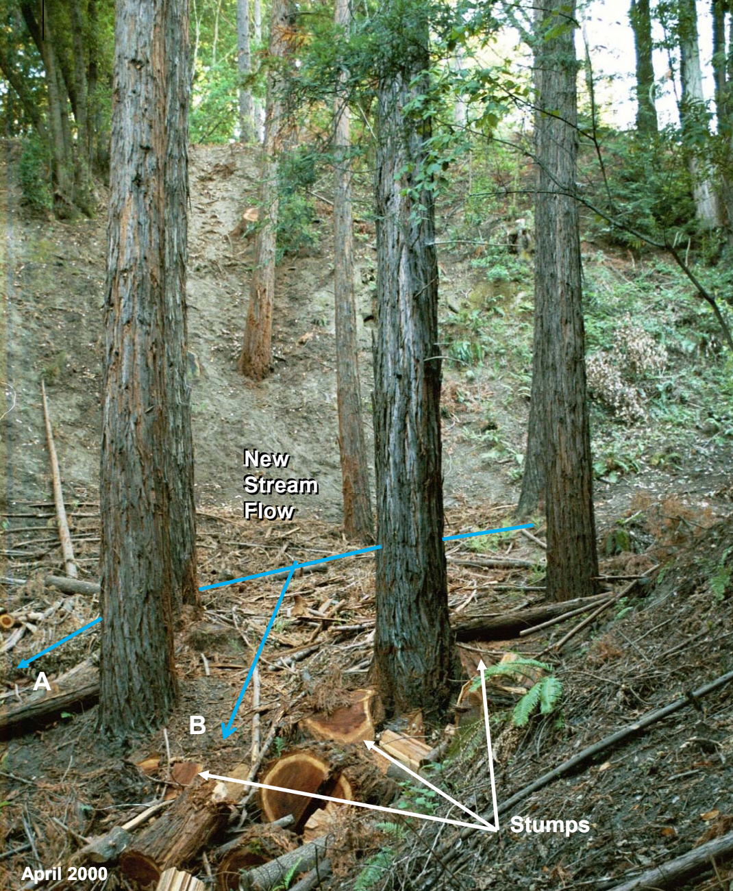
As you can see on the left, I broke the flow into two streams, meaning that the total energy hitting any one spot is greatly reduced. Flow "A" is a great deal lower in slope which thus reduces water velocity. Flow "B" smacks headlong into a stump, which being redwood will last a good long time, especially because it will re-sprout new trees. Because of the slope, I don't expect much deposition here.
