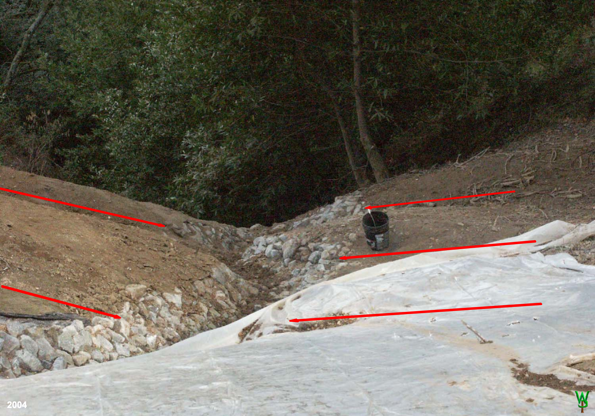
The arrows indicate the alternating benches to catch and redirect sheet wash to the channel. The plastic was not only to preclude rain impingement and sheet wash but it was part of a multivariable revegetation experiment. Then it rained...
