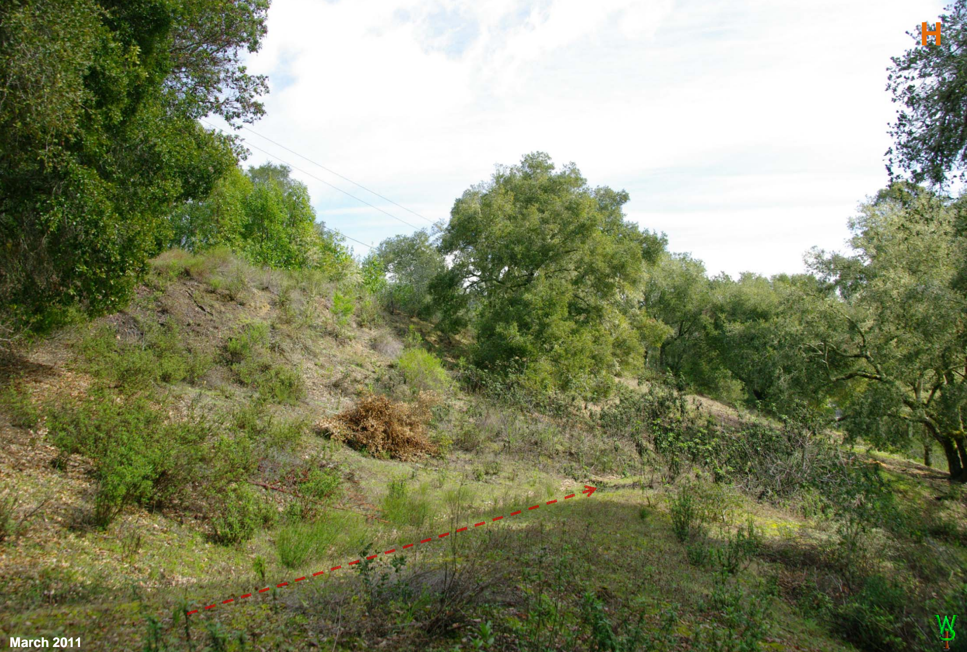
The Sand Hill Road I added (red line) was not optional; it was backup drainage for the driveway in case a culvert plugged, and to protect repairs below that would be subject to slope failure without it. I also needed the fill material. Today, I wouldn't call it picturesque but it is one of the most species-rich and complex parts of the property, supporting many plants that one would prefer not to have elsewhere.
