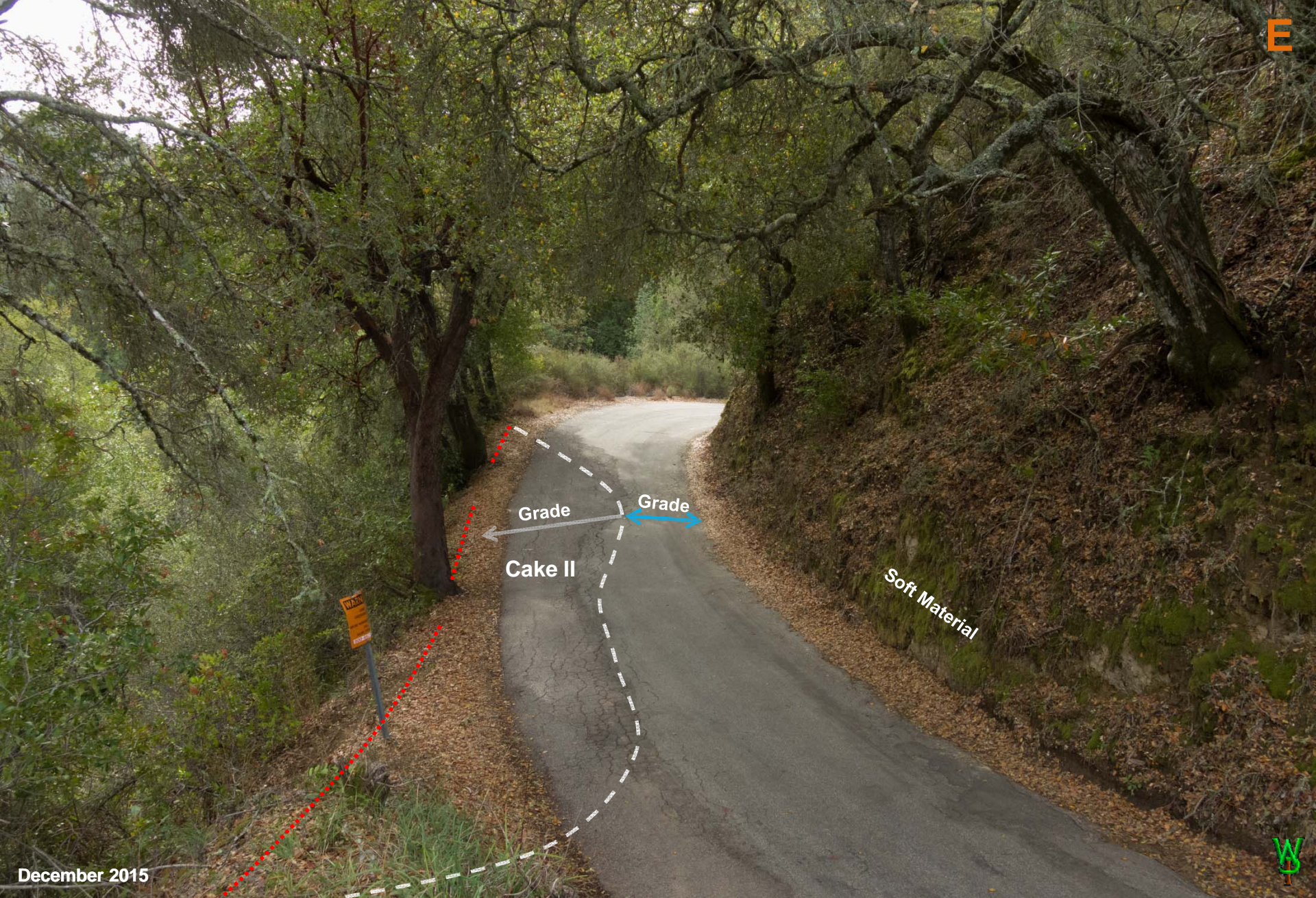
This is a look from the “bump” on the prior slide. With the trees growing in soft material leaning out over the road, it is only a matter of time until one falls, bringing a chunk of dirt with it. That will fill the rest of the drainage “ditch” and send the runoff over the edge and down the headwall . Needless to add, if the trees leaning from atop said headwall go down, they could close the road as well.
