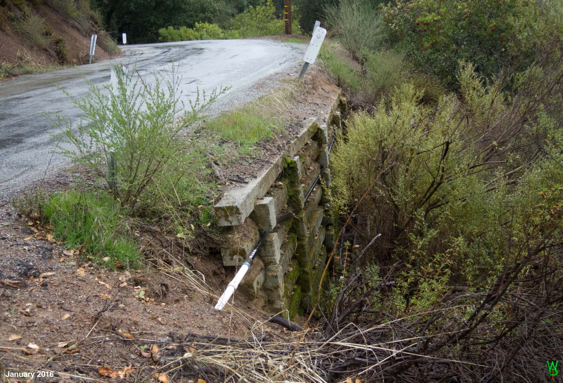
The usual fix for small Type I failures is called a “crib,” basically digging out the cake, making a box with a flat floor on a “stable” substrate, and filling it with rock. Sometimes it is done with concrete “Lincoln logs” and large gravel like you see here. Note: The pipe is the main water supply for nearly 70 homes, many without water storage adequate to fight a fire.
