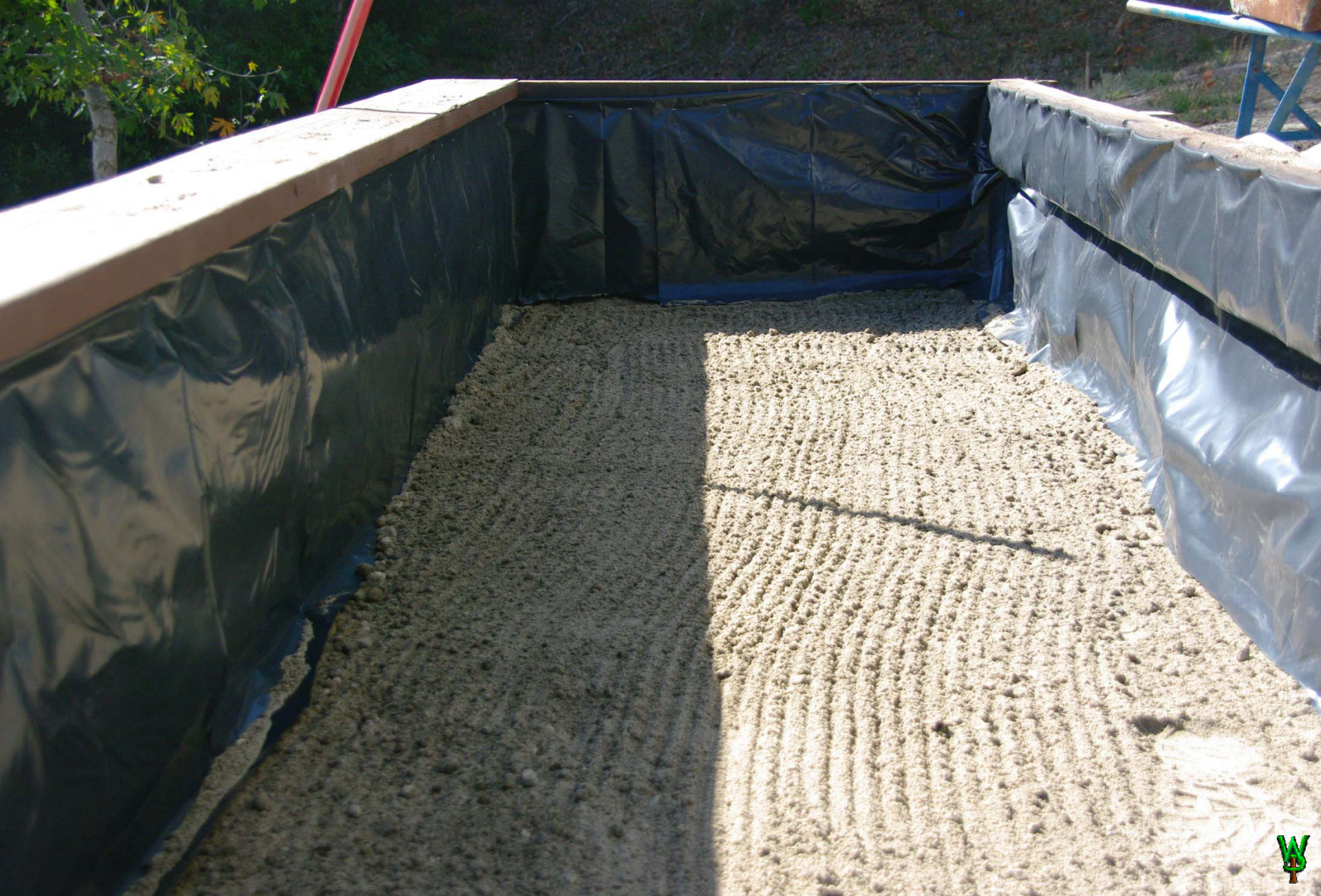
Filter fabric was put on the rock (I would use MiraDrain® today and gain a couple of inches of depth). Then the side walls were lined with doubled 6 mil black polyethylene. This retains moisture in the soil and protects the wood from rot. Sand was put over the filter fabric so that it won't clog. I later protected the top edge with a 1/8" polyethylene "bender board" screwed to the wall with oversized washers.
