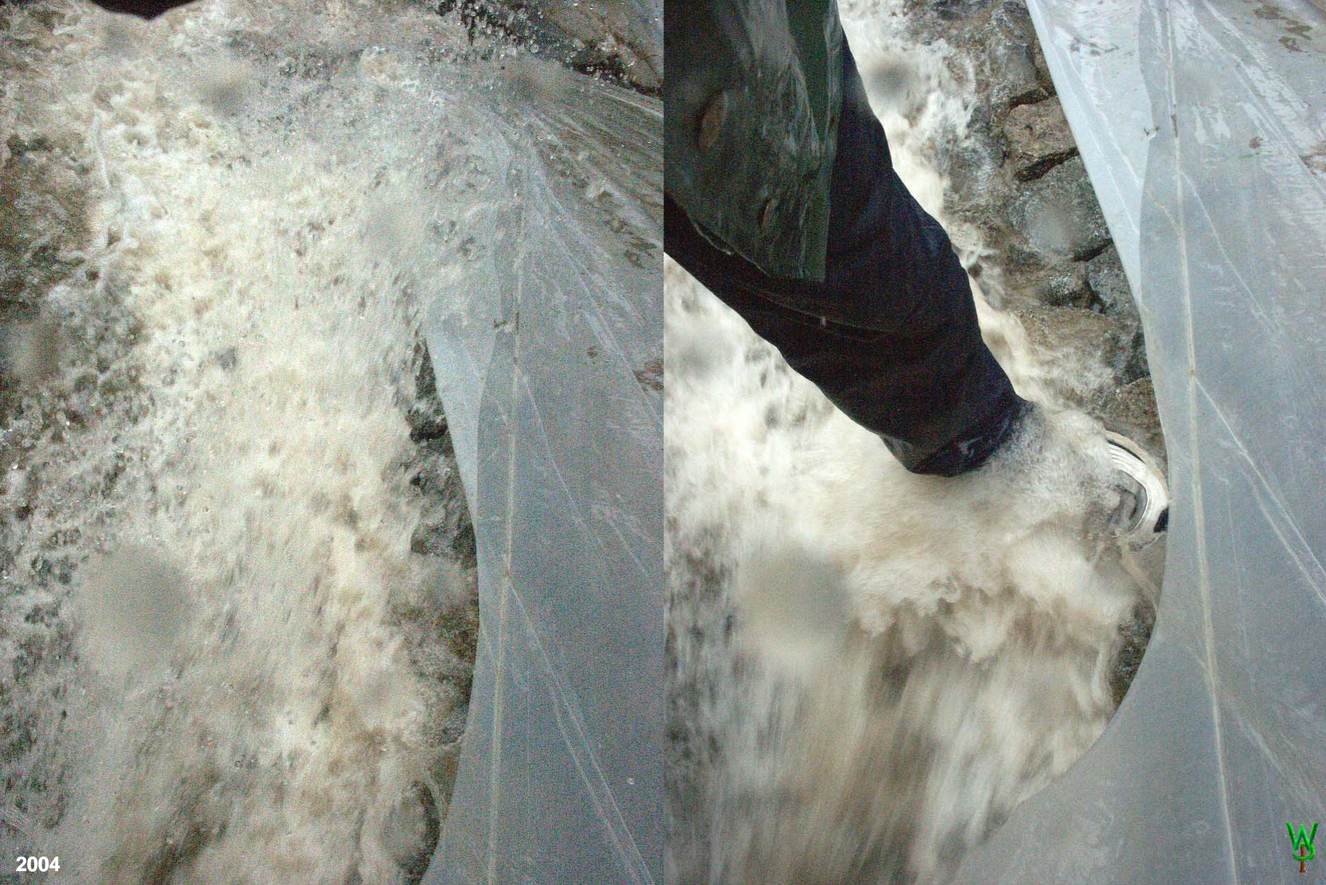
This is when one gets to do the final tweaking. It is very hard to predict how the flow will behave when it exits a pipe. So I waited before dry-setting the rock around the outlet until a storm came to know exactly where and how to adjust for splashing. In this case it only took a couple of hours to reshape the surface.
