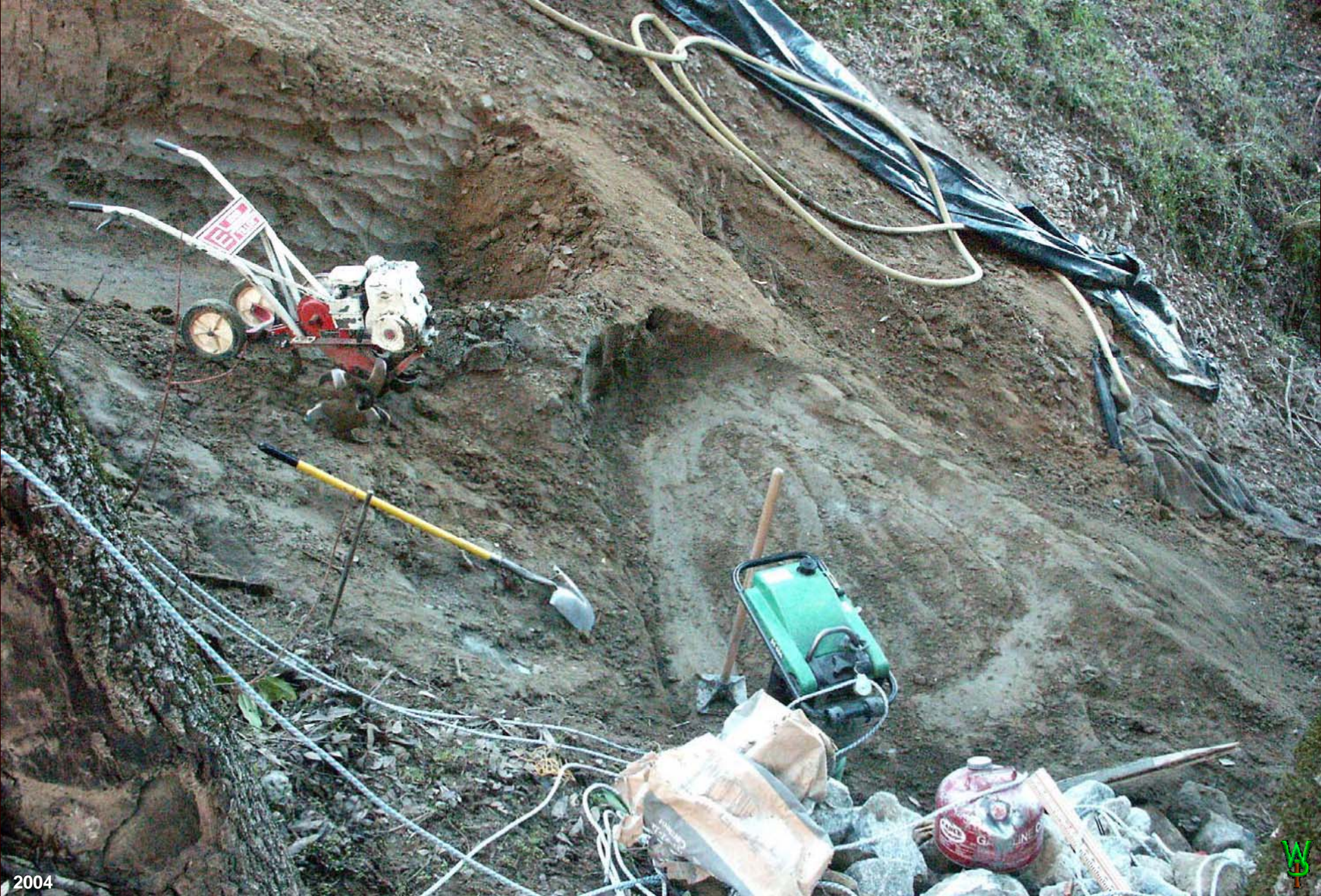
In parts of this project I used the equivalent of a half-sack mix of cement in the soil to reinforce the structure to simulate the attributes of the parent rock and withstand tunneling by ground-squirrels without caving in. It is steep here. Interestingly, the grasses seem to prefer this cemented fill compared to the parent material.
