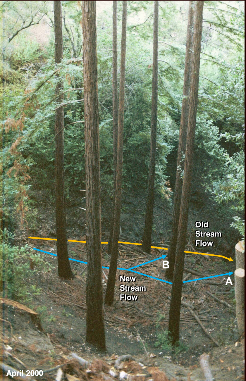
As you can see on the left, I broke the flow into two streams, meaning that the total energy hitting any one spot is greatly reduced. The run-out slope "A" is a great deal lower which also reduces water velocity. Flow "B" smacks headlong into a stump, which being redwood will last a good long time, especially because it will re-sprout new trees. Because of the slope, I don't expect much deposition here.
