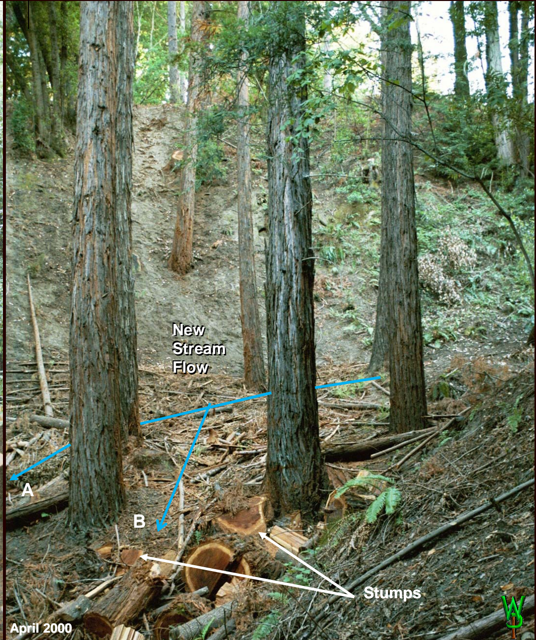
As you can see on the left, I broke the flow into two streams, meaning that the total energy hitting any one spot is greatly reduced. The run-out slope "A" is a great deal lower which also reduces water velocity. Flow "B" smacks headlong into a stump, which being redwood will last a good long time, especially because it will re-sprout new trees. Because of the slope, I don't expect much deposition here.
