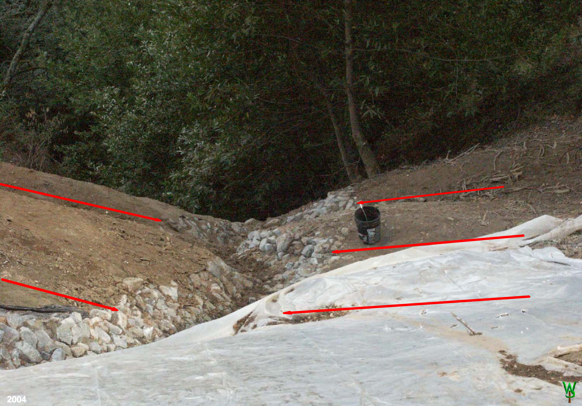
It is steep here. The arrows indicate the alternating benches to catch and redirect sheet wash to the channel. The plastic was not only to preclude rain impingement and sheet wash but was part of a multivariable revegetation experiment. Then it rained...
