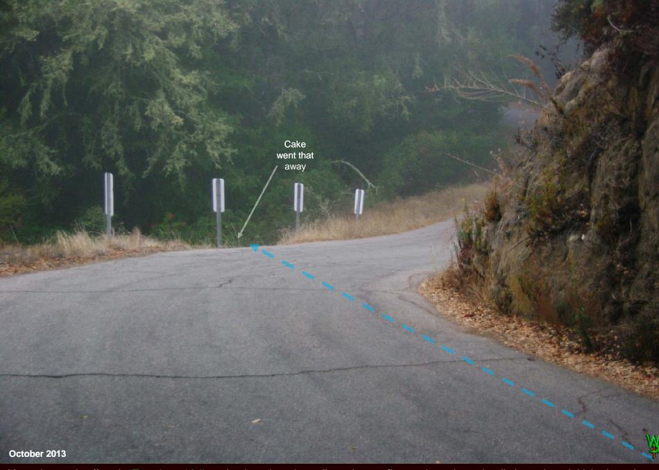
Here, the road suffered a Type I road failure: In-sloped grades collected water flow and ran down the ditch to where it kicked out due to accumulated sediment. Then it ran across the surface away from the ditch, hit the corner (above), kept going, and just took the cake.
