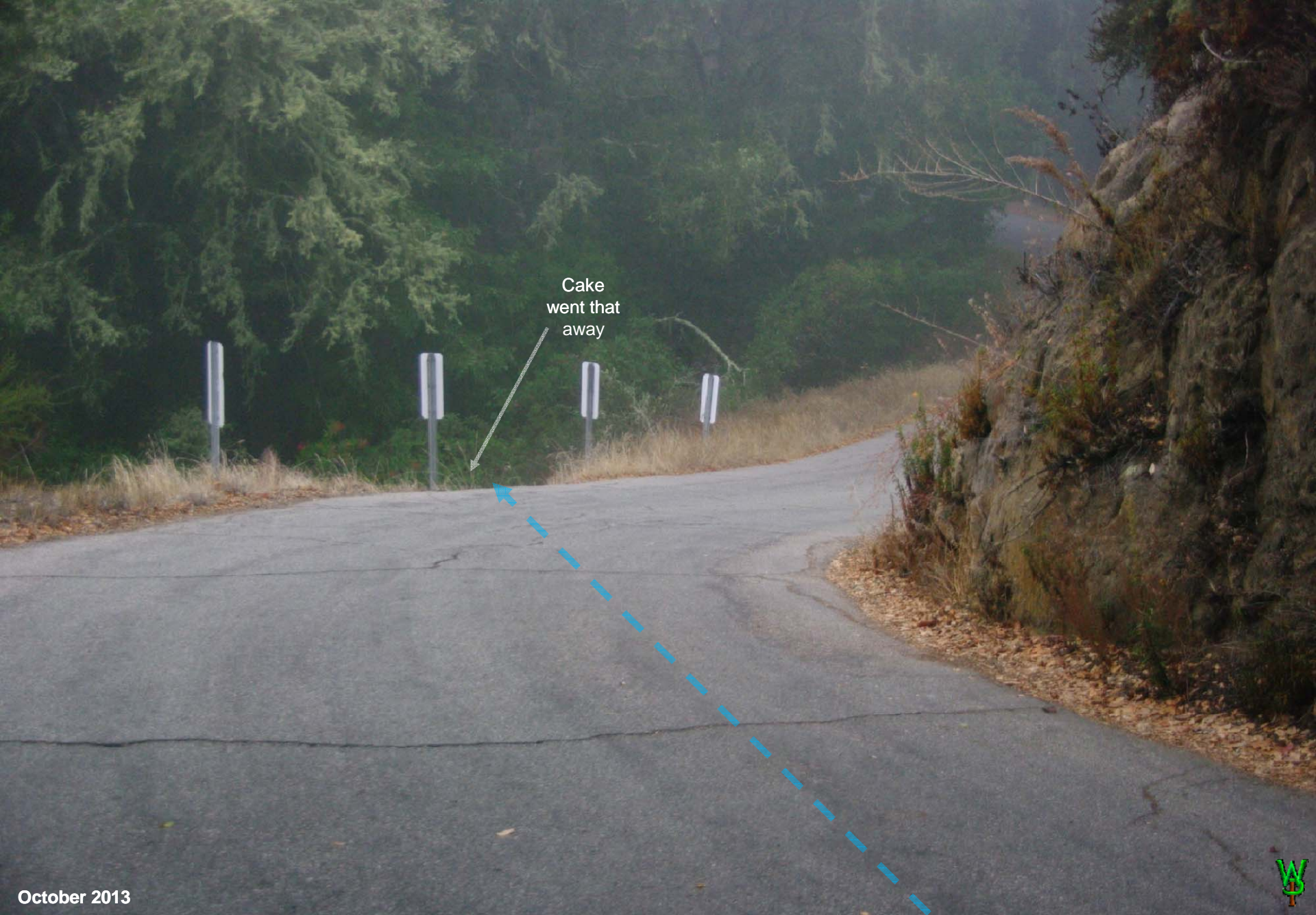
The spot suffered a Type I road failure: In-sloped grades collected water flow and ran down the ditch to where it kicked out due to accumulated sediment. It then ran down the surface away from the ditch, hit the corner (above), kept going, and just took the cake.
